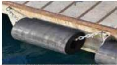
Gambar 5. Fender tipe slinder (Sumber: Azizul, 2019)
